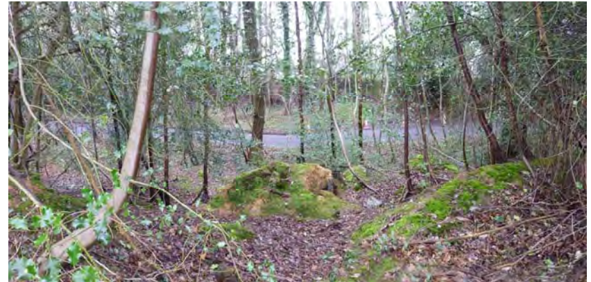
Embankment at the site boundary with Coos Lane
