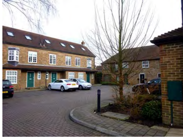
Infill development - Caffyns Cottages
