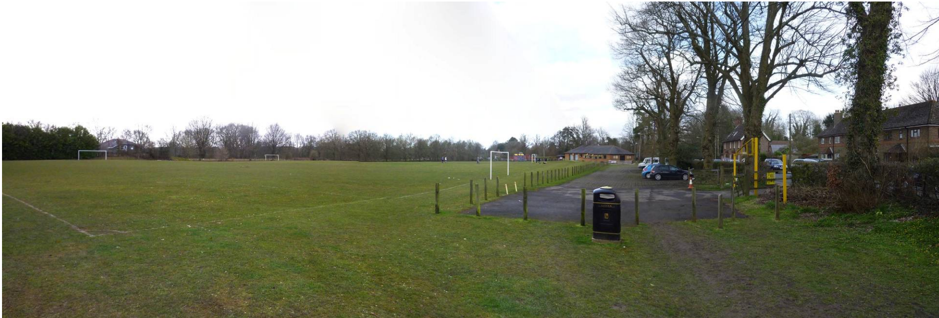
view looking north showing access roadway, parking and pavilion building
